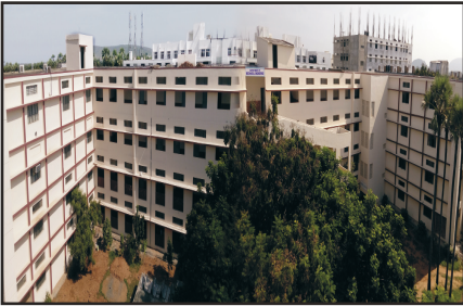
Mechanical Engineering (F-Block)
