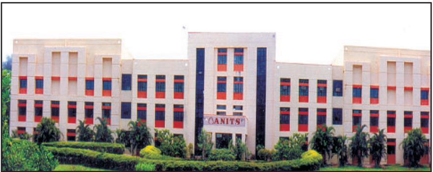
Administrative Block (A - Block)
