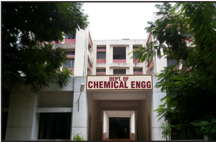
Chemical Engineering (D-Block)
