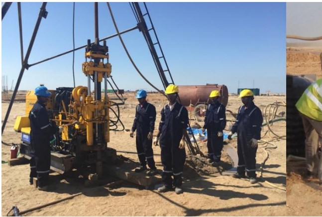
Figure 4: Soil investigation using borehole drill rigs
