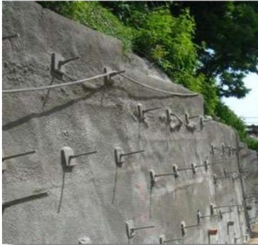
Fig.1.Soil Nailing
