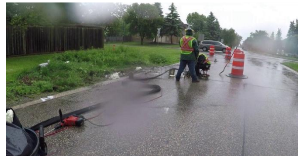
Fig.3 precast slabs under sealed with polyurethane foam
